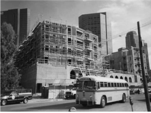
Figure 2. Apartment complex utilizing FRTW studs.
