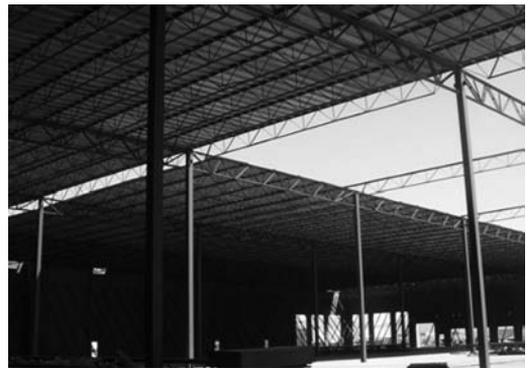
Figure 1. FRTW panelized roof system.
